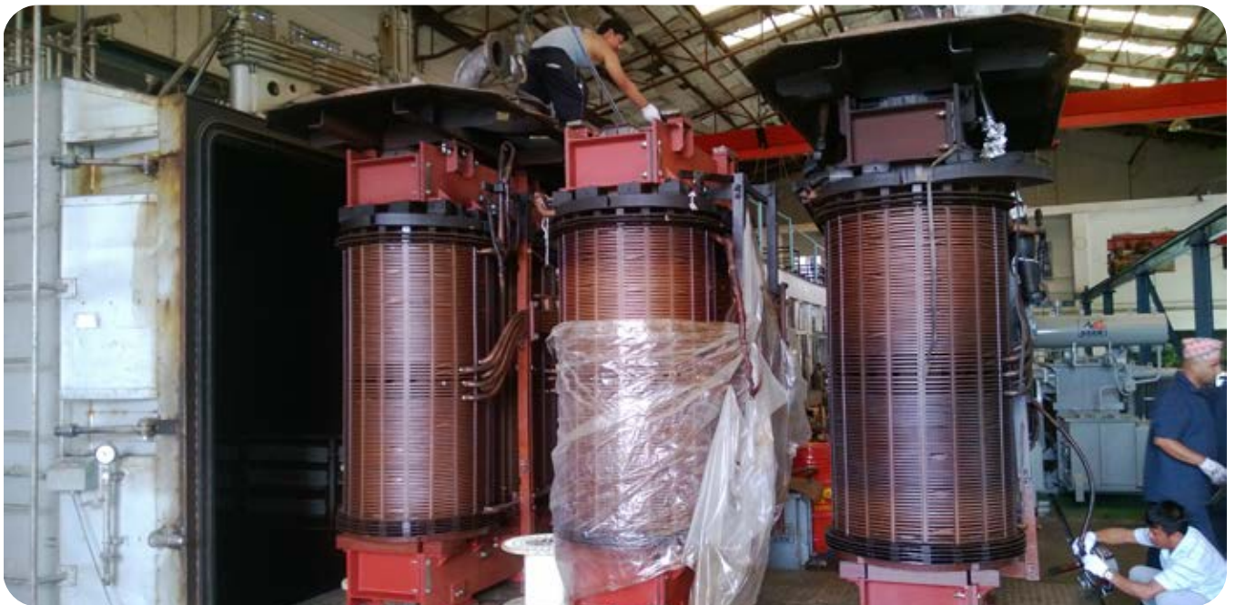
12.6 MVA 132/6.6 kV Power Transformer being repaired Kulekhani-II Hydropower
