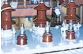
HV bushing with terminal connectors
